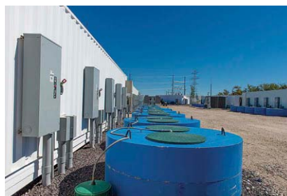
WHIRLING WATTAGE: Beacon Power built a 20-megawatt plant in Hazle, Pa. It started regulating grid frequency in July 2014.
